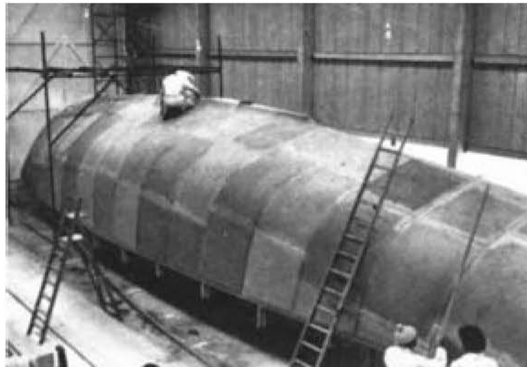
Figure 16 Foam sheets on framework
