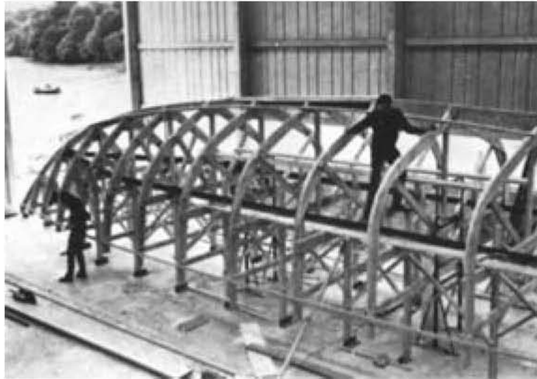
Figure 15 Wooden framework for mouldless construction
